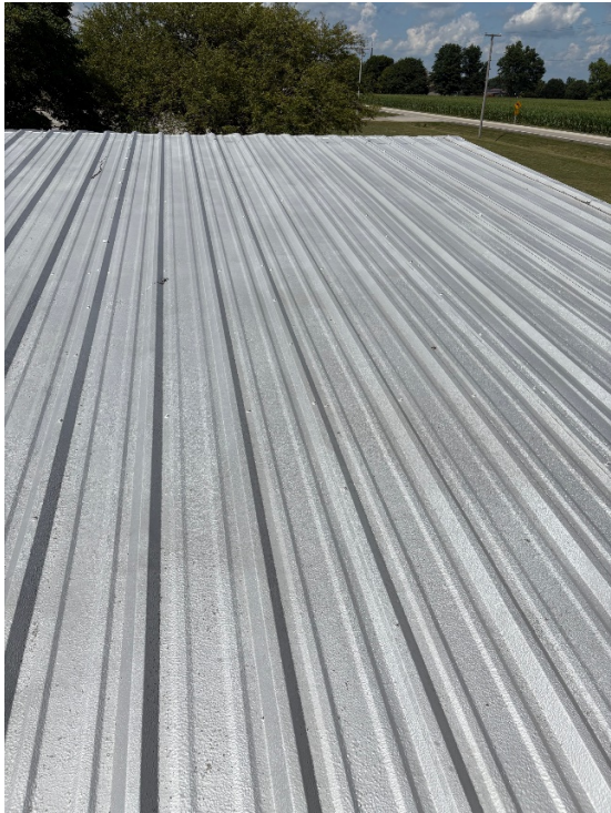
Original roof lap seam, exposed fasteners 12" rib spacing always verify
