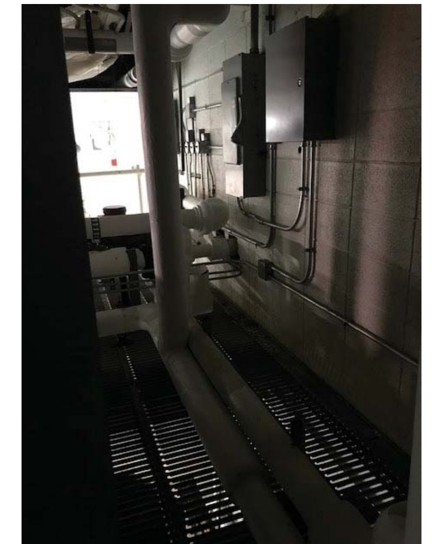
SOUTH END LOOKING EAST
