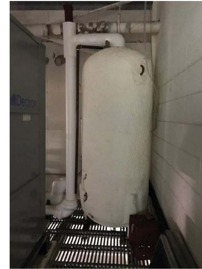
WEST LOOKING SOUTH
