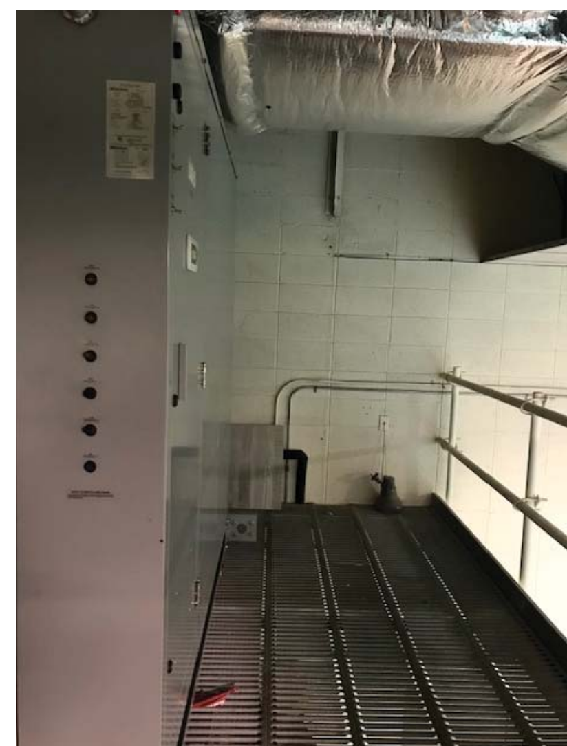
NORTH END OF PLATFORM
