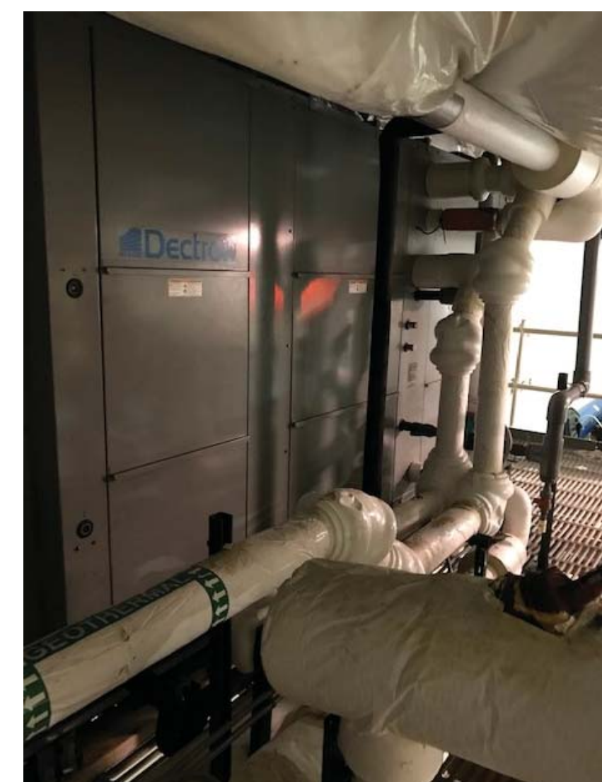
EAST SIDE LOOKING NORTH
