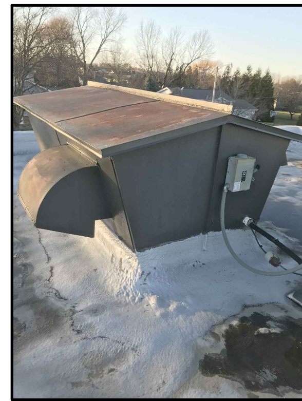
PC DISTRICT OFFICE NORTH ROOF PHOTO D
