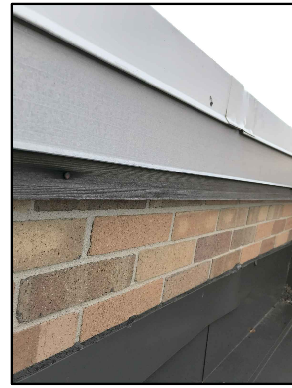
PCHS 1972 ADDITION ROOF PHOTO M
