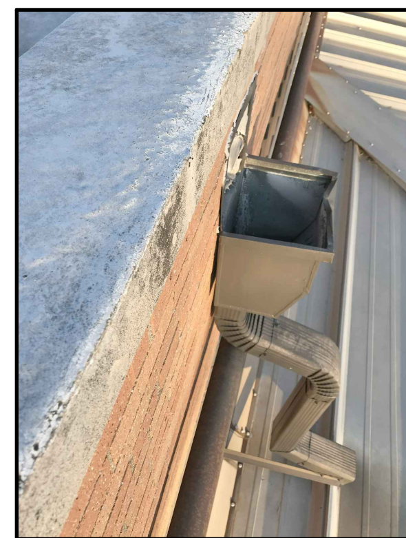
PC DISTRICT OFFICE NORTH ROOF PHOTO I
