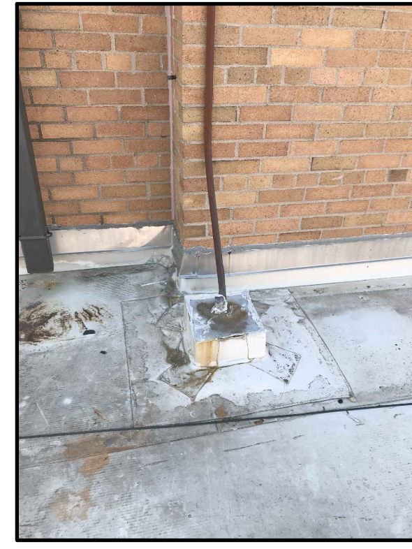
PCHS 1972 ADDITION ROOF PHOTO F
