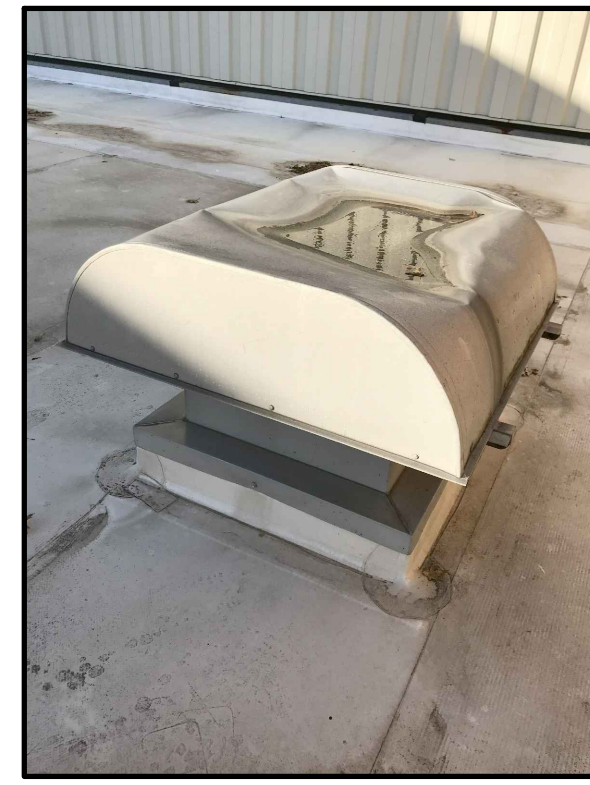
PCHS 1972 ADDITION ROOF PHOTO I
