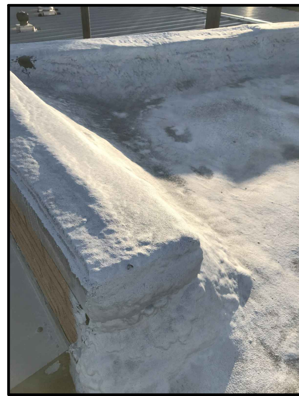
PC DISTRICT OFFICE NORTH ROOF PHOTO A
