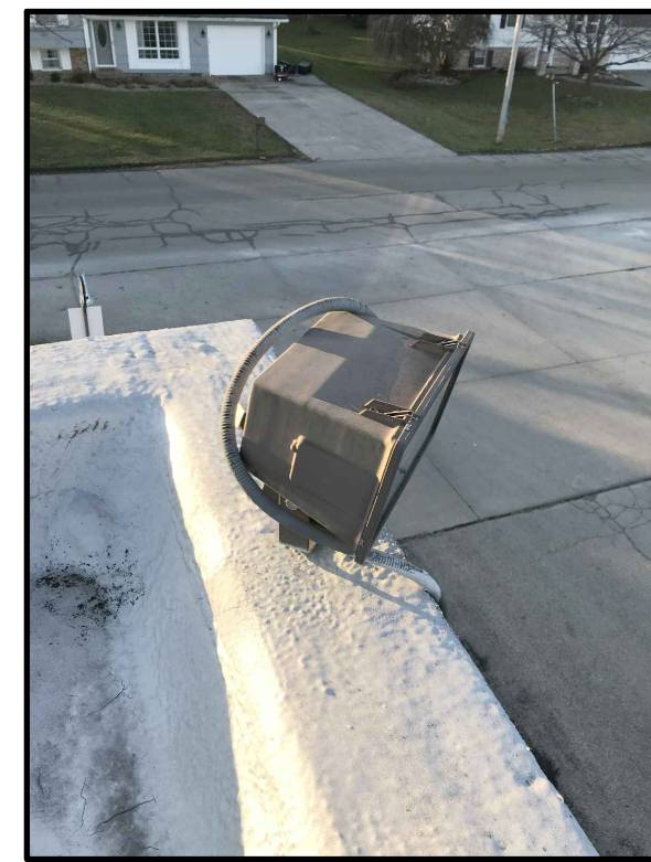
PC DISTRICT OFFICE NORTH ROOF PHOTO F
