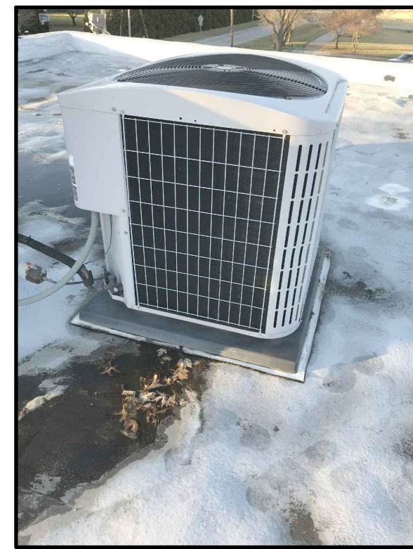
PC DISTRICT OFFICE NORTH ROOF PHOTO C
