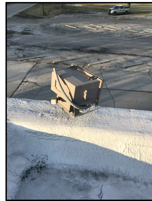
PC DISTRICT OFFICE NORTH ROOF PHOTO E
