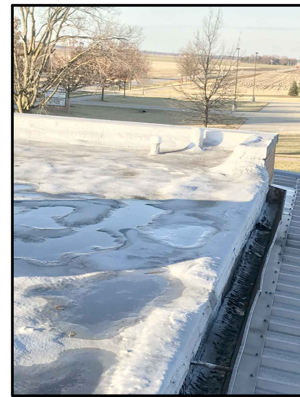
PC DISTRICT OFFICE NORTH ROOF PHOTO B
