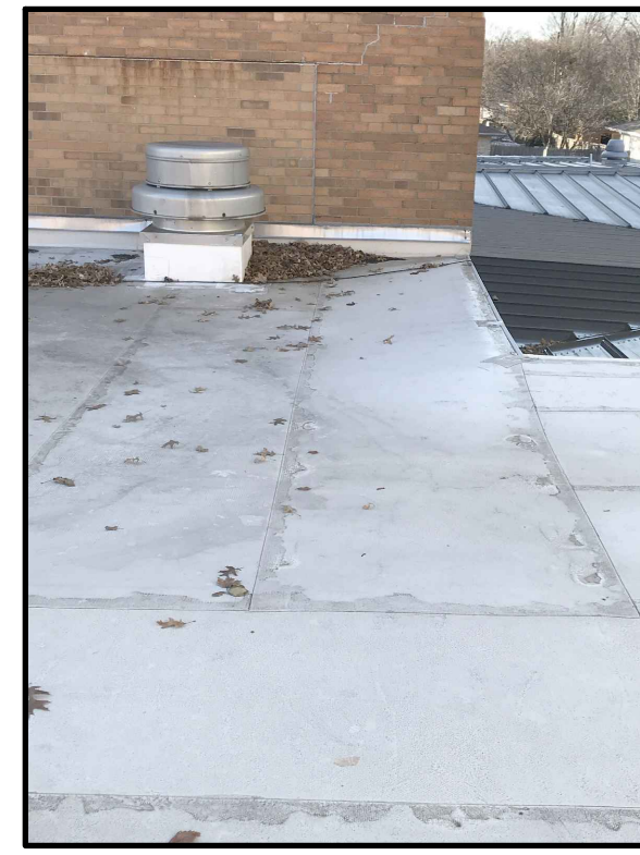
PCHS 1972 ADDITION ROOF PHOTO K
