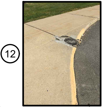
PEPPER RIDGE PAVING (12)
