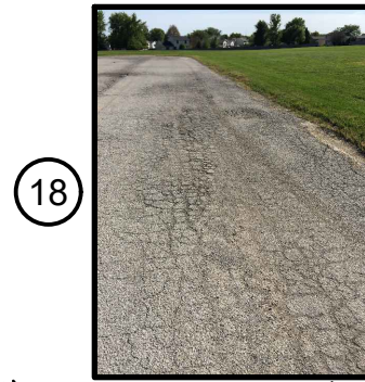
PEPPER RIDGE PAVING (18)
