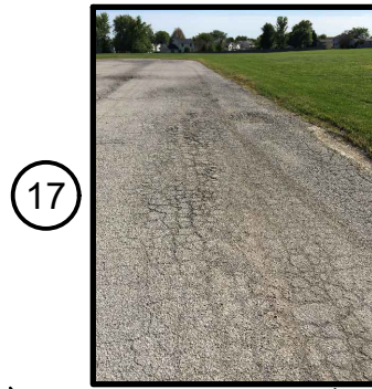
PEPPER RIDGE PAVING (17)
