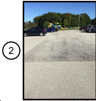
PEPPER RIDGE PAVING (2)
