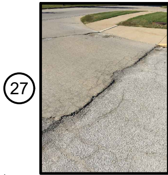
PEPPER RIDGE PAVING (27)
