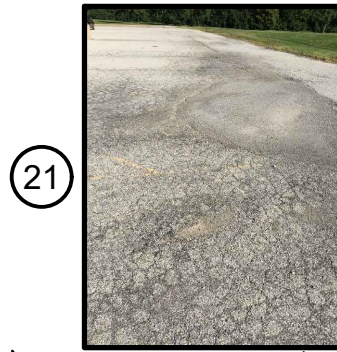
PEPPER RIDGE PAVING (21)
