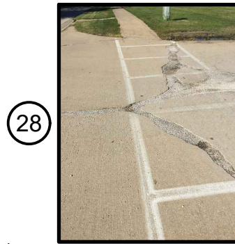
PEPPER RIDGE PAVING (28)
