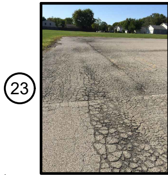
PEPPER RIDGE PAVING (23)
