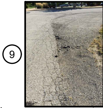
PEPPER RIDGE PAVING (9)
