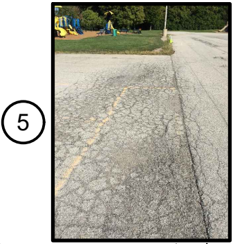
PEPPER RIDGE PAVING (5)
