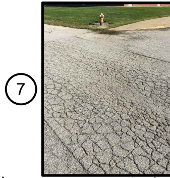
PEPPER RIDGE PAVING (7)
