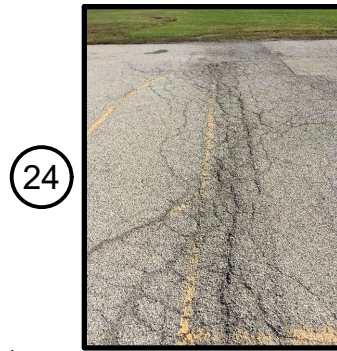
PEPPER RIDGE PAVING (24)
