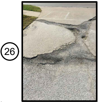
PEPPER RIDGE PAVING (26)
