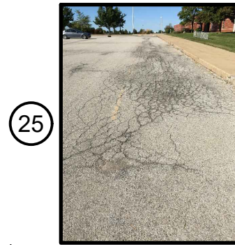
PEPPER RIDGE PAVING (25)
