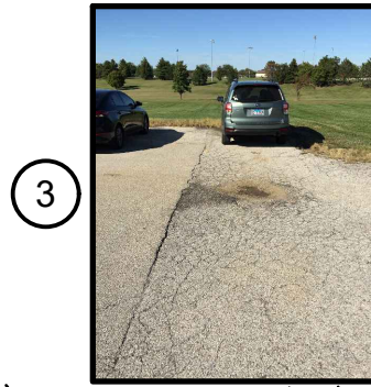
PEPPER RIDGE PAVING (3)
