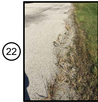
PEPPER RIDGE PAVING (22)
