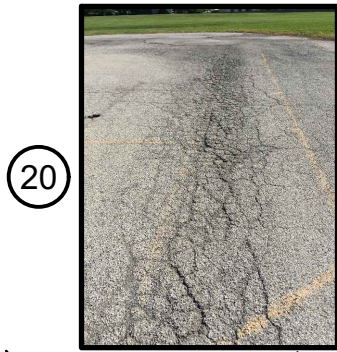
PEPPER RIDGE PAVING (20)
