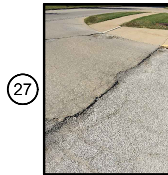
PEPPER RIDGE PAVING (27)
