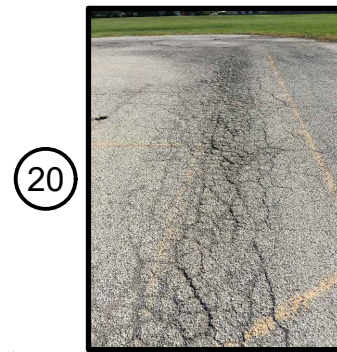
PEPPER RIDGE PAVING (20)
