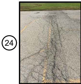
PEPPER RIDGE PAVING (24)
