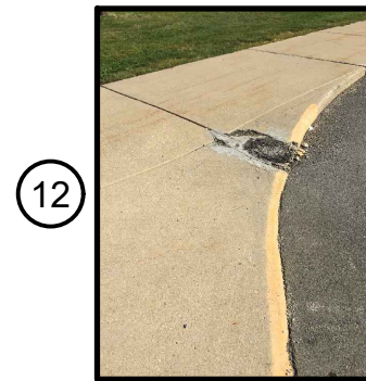
PEPPER RIDGE PAVING (12)
