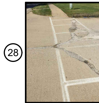
PEPPER RIDGE PAVING (28)
