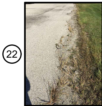
PEPPER RIDGE PAVING (22)
