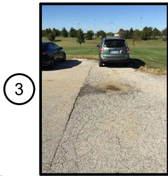
PEPPER RIDGE PAVING (3)
