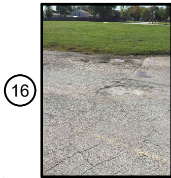
PEPPER RIDGE PAVING (16)
