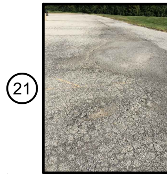
PEPPER RIDGE PAVING (21)
