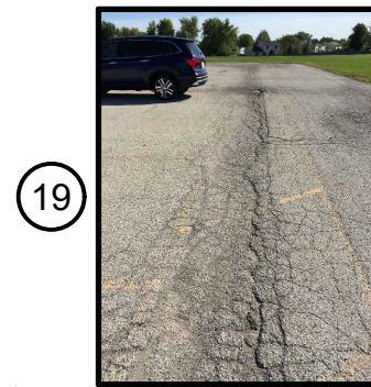
PEPPER RIDGE PAVING (19)
