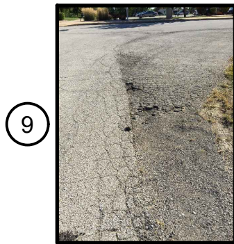
PEPPER RIDGE PAVING (9)
