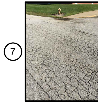
PEPPER RIDGE PAVING (7)
