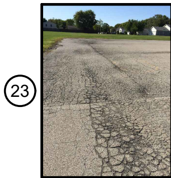
PEPPER RIDGE PAVING (23)
