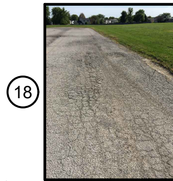
PEPPER RIDGE PAVING (18)
