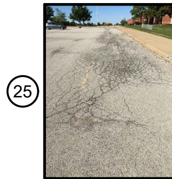
PEPPER RIDGE PAVING (25)
