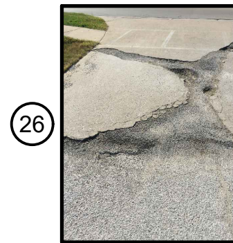
PEPPER RIDGE PAVING (26)
