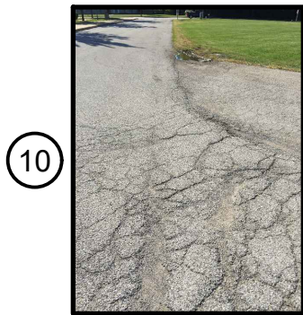
PEPPER RIDGE PAVING (10)
